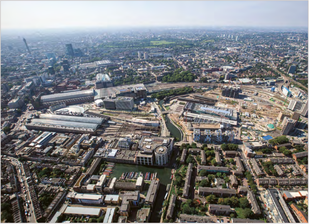
Aerial picture of the development site
