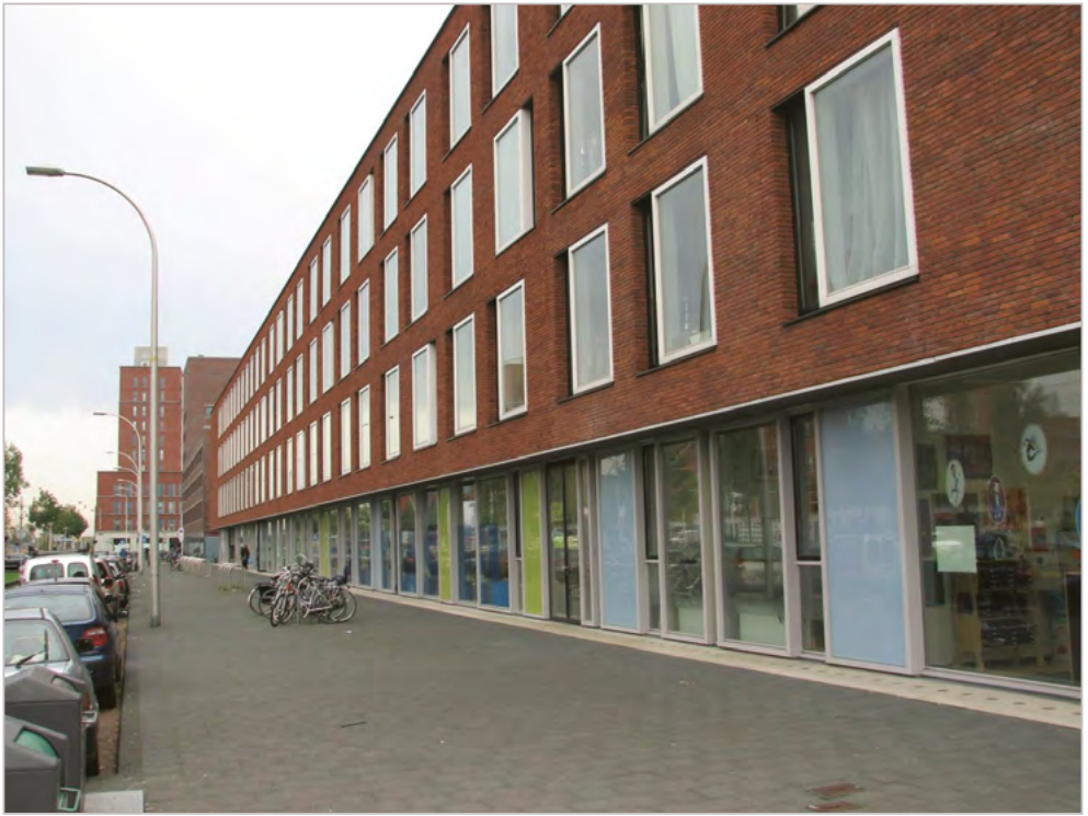
Primary school in the child rich newly built neighbourhood Ypenburg (The Hague) that over twenty years easily can be transformed for other purposes
