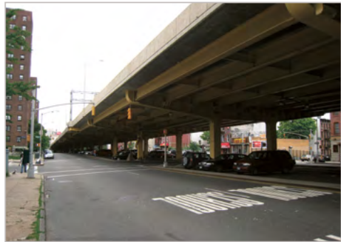
Elevated highway in New York, Williamsburg
