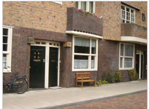
Residential plinth in Amsterdam
