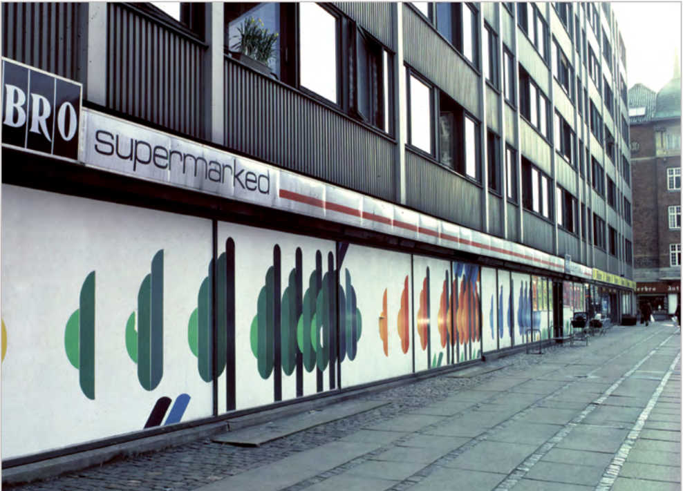
Closed façades with uniform functions: passive and boring
