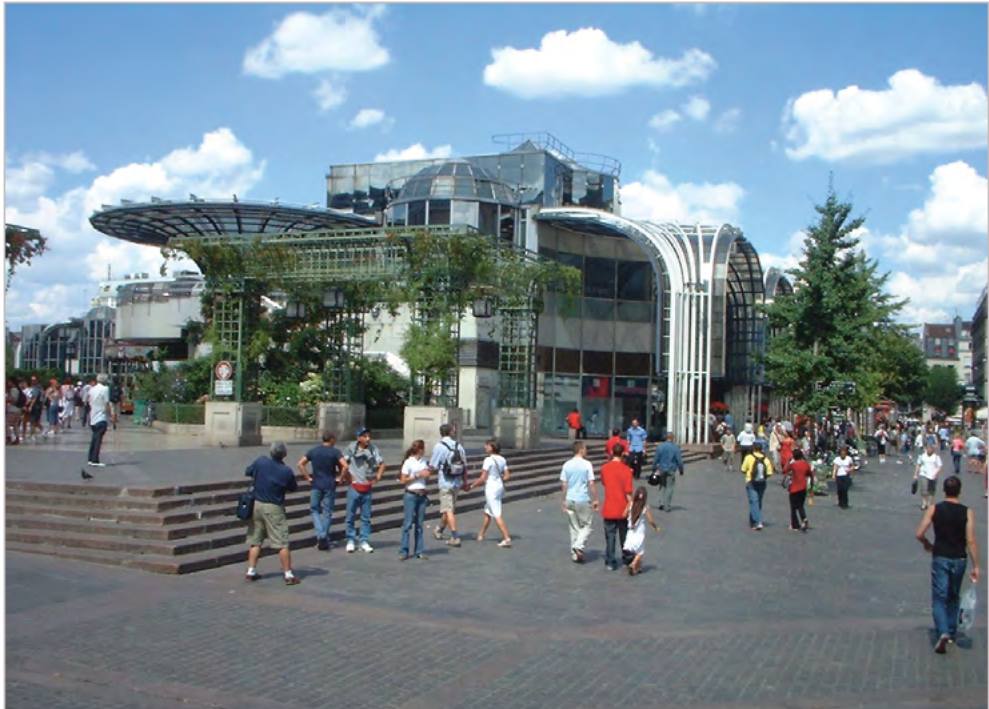
Forum Les Halles, Paris: constructed in 1977, demolished in 2010 and to be replaced by a new Forum
