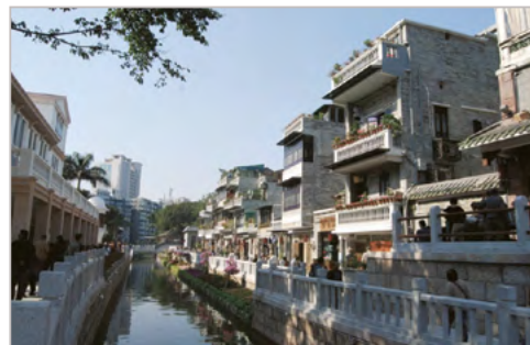
A street and water channel after reconstruction
